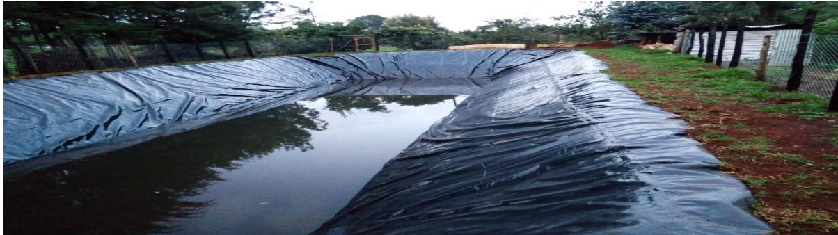
Plate 2: A water reservoir in Igwamiti ward, Laikipia west Sub County. Sources: field data (November, 2019)
