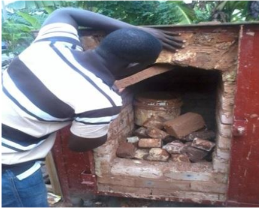
Plate 39: Making the arch of the kiln.
