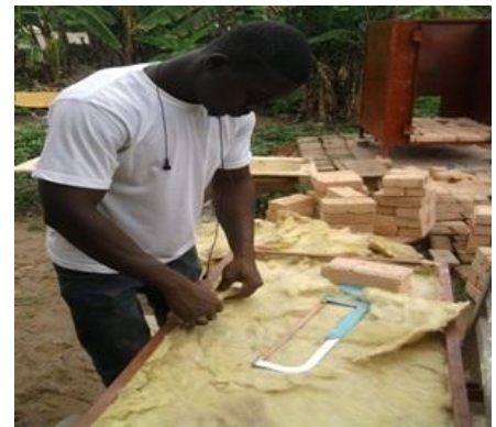
Plate 36: Lining the inside of the door with fibre
