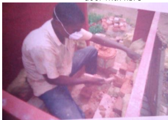
Plate 38: Arrangement of refractory bricks in the kiln
