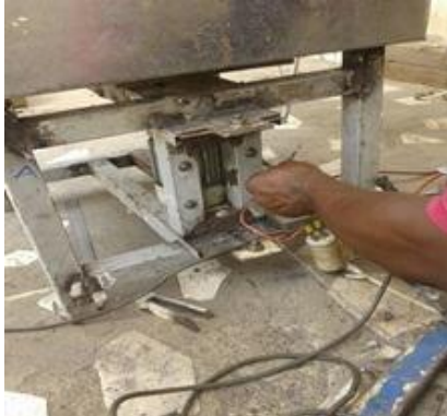
Figure 21: Rewiring electric motor
